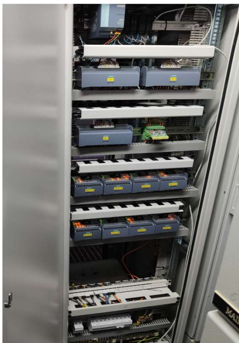
The control rack replaced with a new PLC-based one
